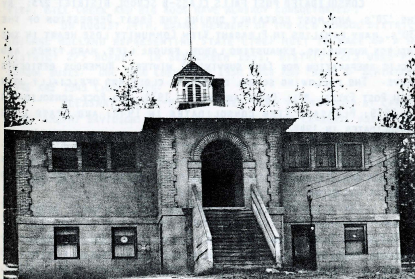
PLEASANT VIEW COMMUNITY ASSOCIATION'S HALL (I.E. THE OLD PLEASANT VIEW SCHOOL HOUSE) AS IT LOOKED AFTER MASSIVE WORK AND CLEAN-UP. CA 1975. LISTED WITH THE IDAHO PRESERVATION COUNCIL AND ON THE NATIONAL REGISTRY. (COMPL. GLEN AND EVA MADISON).
